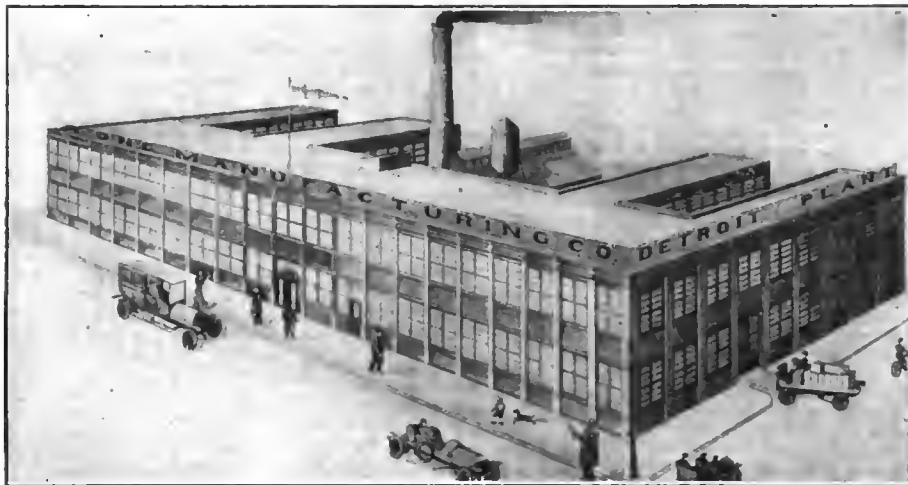
New Long Radiator Plant at Detroit, Mich.
